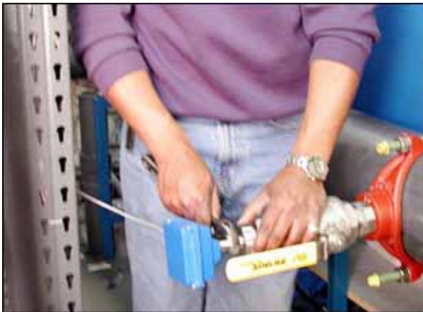
1. Loosen compression fitting
